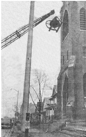
Removing the bells from the old church building
